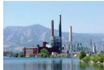
Valmont Power Plant ~200 MegaWatts Boulder, CO
